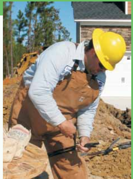
The trend in new service construction is for underground installation.
