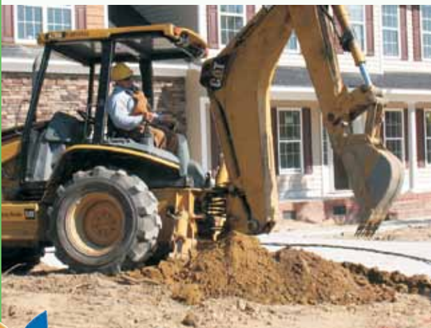
Crews installed 34.5 miles of underground service in 2008.
